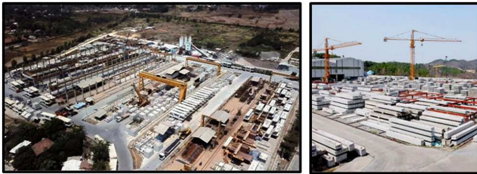
FIGURE 2. Situation map for precast concrete product stockyard
